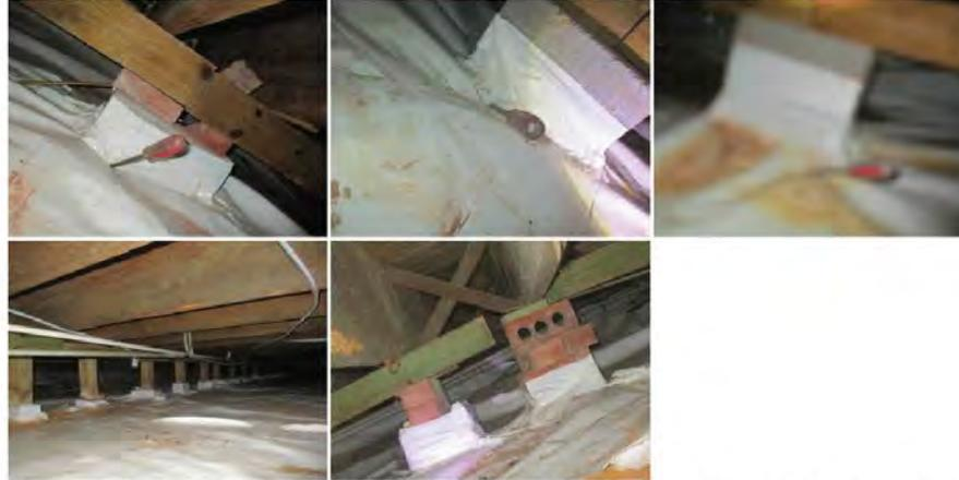
3. Main Crawl Space Moisture Penetration: Left outside wall - There are signs of past moisture intrusion along the left side wall. This can lead to moisture damage to the floor system and organic growth on the wood. A qualified contractor is recommended to evaluate and estimate repairs
