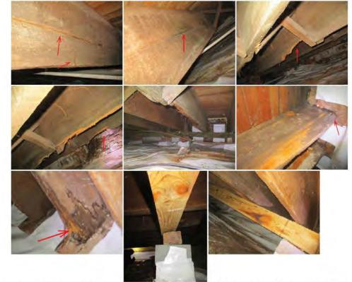
Columns: Block and Brick piers - Multiple support posts and block piers have been installed to help support the floor system. If any of the supports are deemed to be structural supports they need proper footings. A qualified contractor is recommended to evaluate and estimate any repairs
