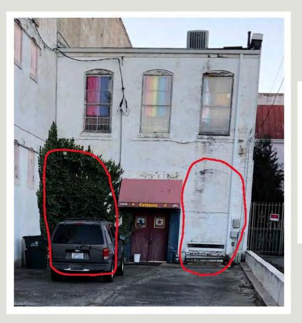
The two lower bricked over windows to be restored and white paint and shrubbery removed to restore and protect the redbrick wall. Bricks to be reappointed as required – \$4000
