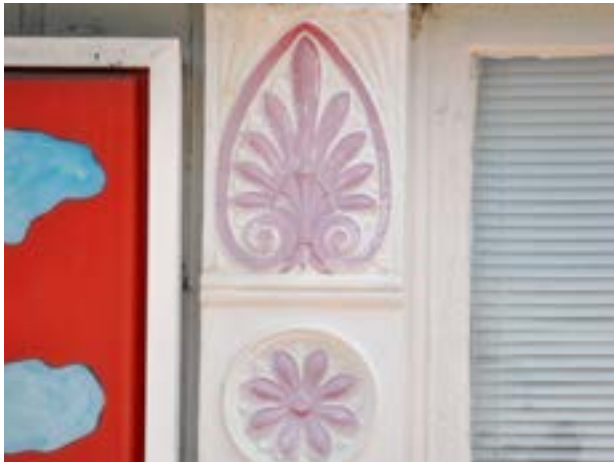
Detailing on Metal Pier
