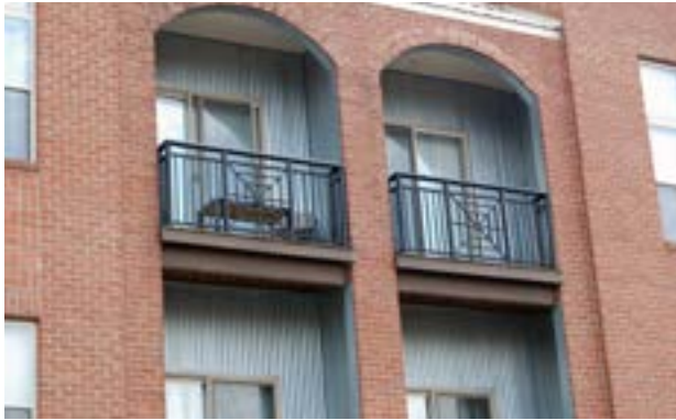
Contemporary balcony using appropriate materials
