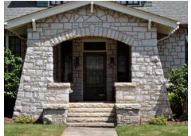
Tapered Stone Columns on Craftsman Entryway
