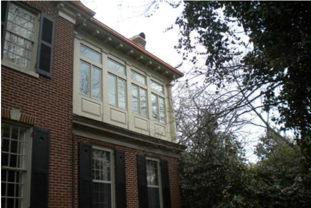
Rear addition over existing garage in West Square Historic District
