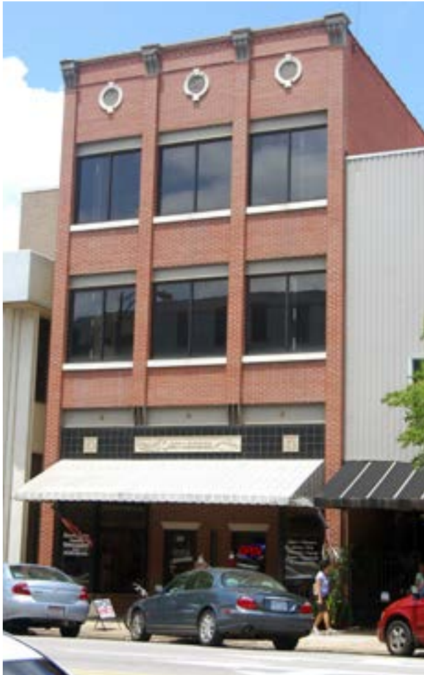
The New Facade on the Oestreicher Building in Downtown Replaced an Inappropriate 60's Era Cladding
