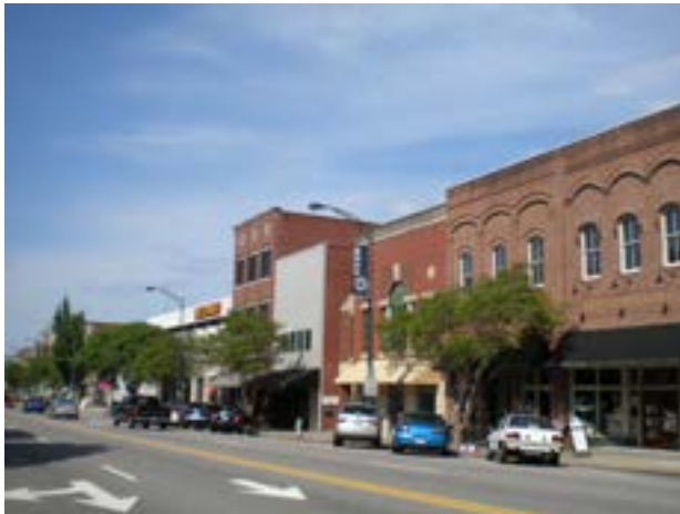
Commercial Architecture in Downtown Salisbury
