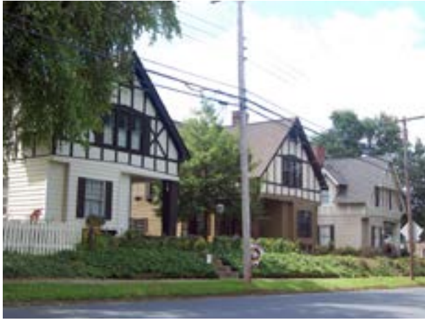
Tudor Revival homes in Ellis Street Graded School District.
