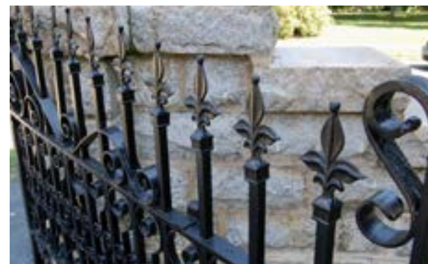
Cast Iron Gate
