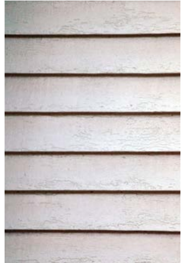
Wood Clapboard Siding Detail
