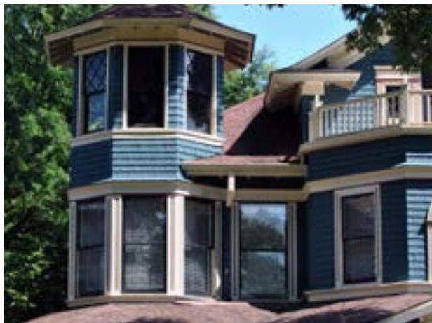
Paint Detail on Historic Home
