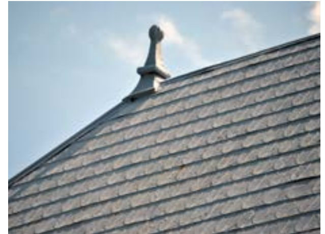
Pressed Metal Roof Detail
