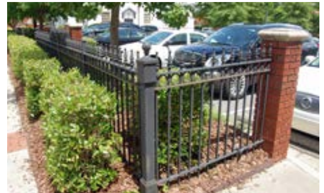
Iron Fencing with Cast Spindles
