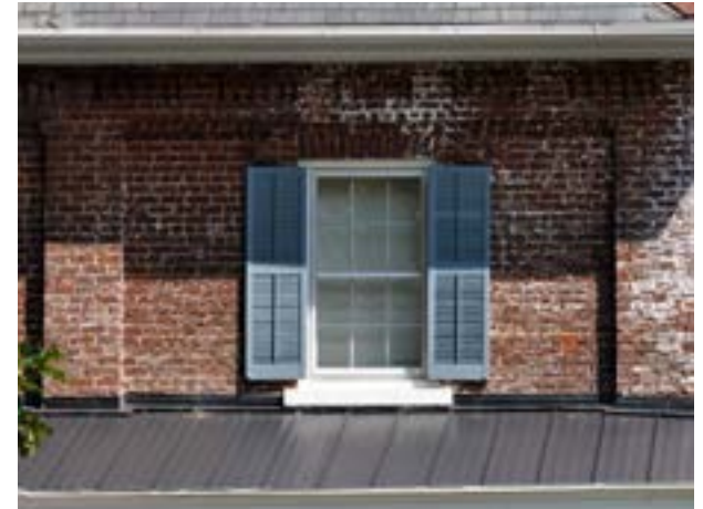
Historic Brick Structure with Paint Removed
