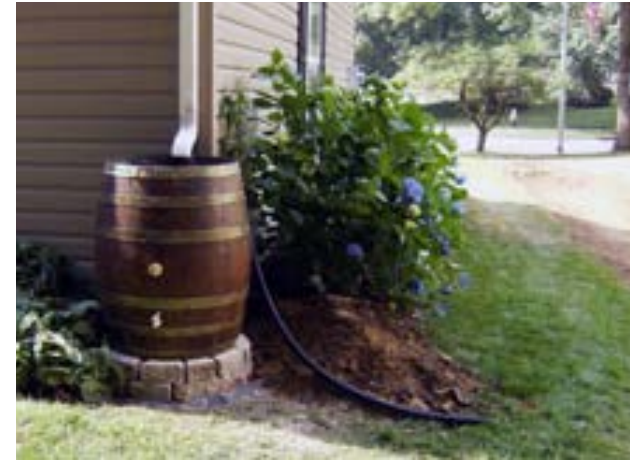
Rain Barrel Water Collection on Residential Structure
