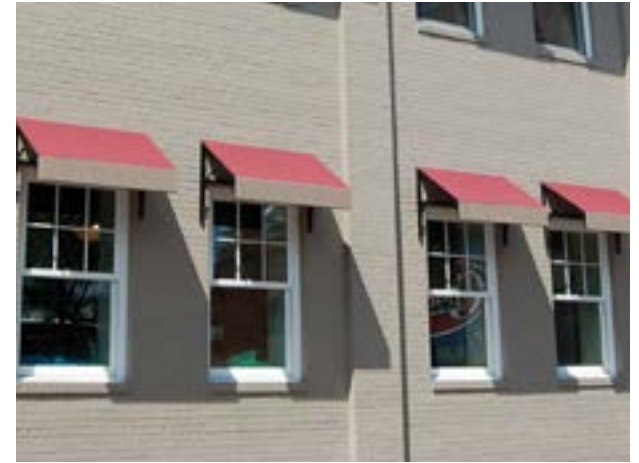
Awnings Applied to Historic Windows
