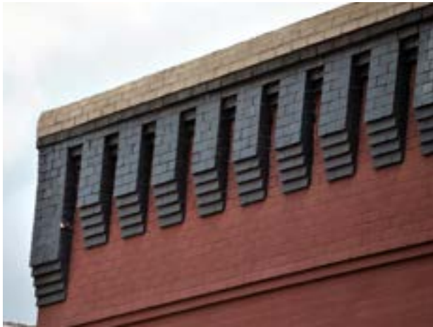
Brick corbelling on facade of 118 E Council Street.
