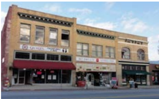
Commercial Architecture in Downtown
