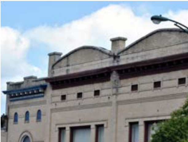
Parapet Walls on Downtown Buildings
