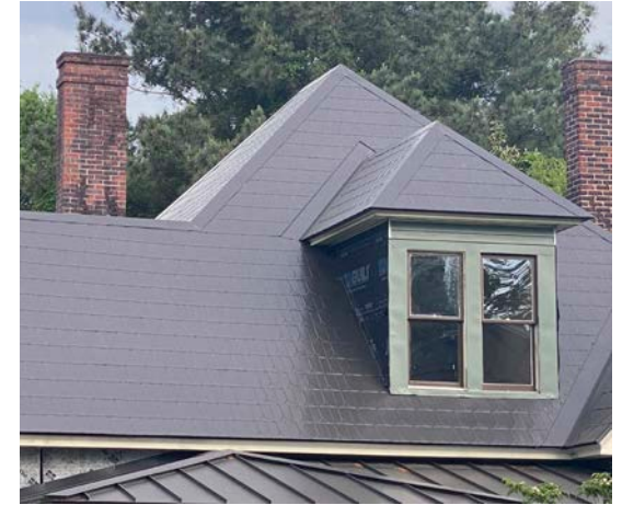
Replacement metal Victorian shingles
