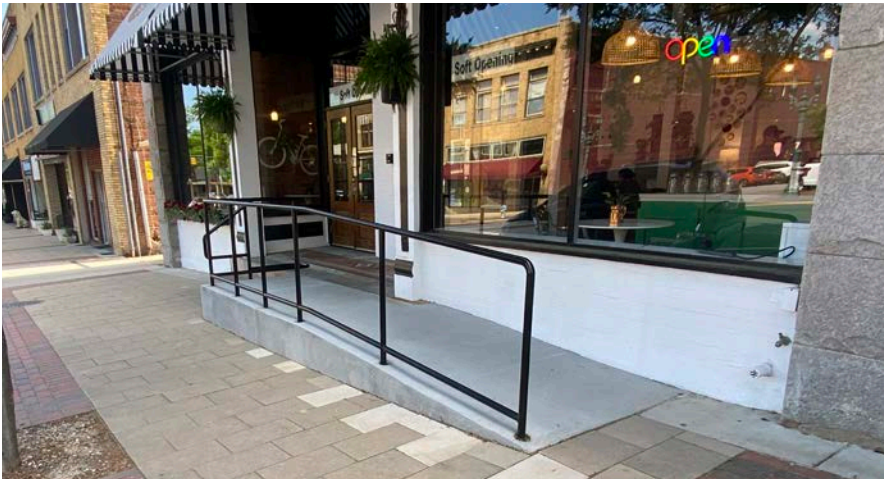
Reversible concrete ramp on commercial storefront
