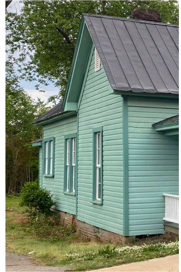
Maintain a sound paint film on wooden siding and windows to prevent damage from sunlight and moisture
