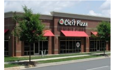
A building and its primary entrance façade shall be oriented toward the street. (5.6.A)
