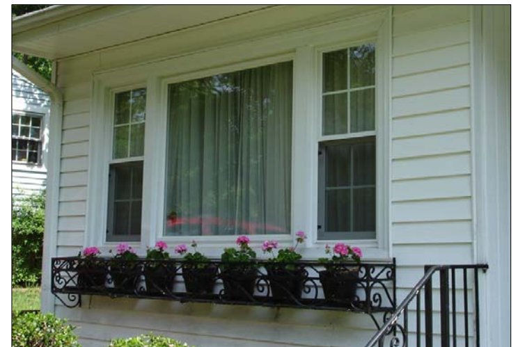
Figure 23: This replacement window appropriately fits within the openings of the original building.
