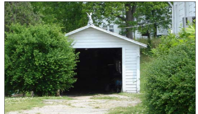
Figure 27: Simple detached garages are encouraged, like this example at 706 West Kerr Street.
