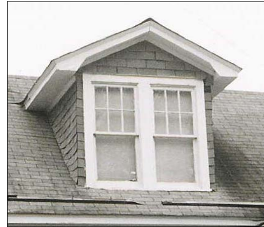
Figure 17: Significant architectural features in Jersey City include porches, overhanging roofs, window detailing, and dormer windows.
