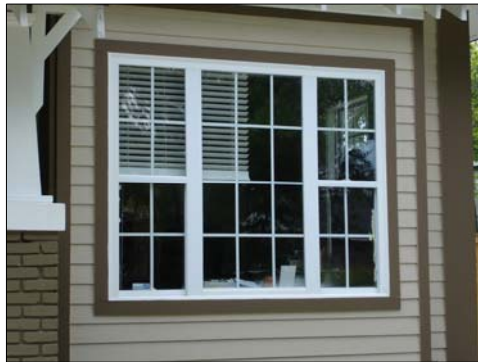
Figure 28: Synthetic materials that complement existing architecture are appropriate.
