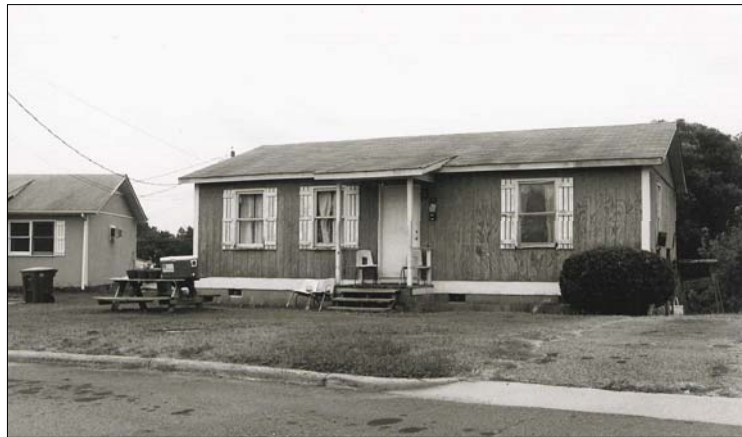
Figure 2: Many non-descript homes contribute nothing to the character nor respect the history of Jersey City.
