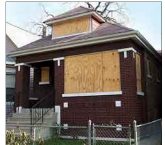
Figure 16: Deteriorated and Boarded-up Home
