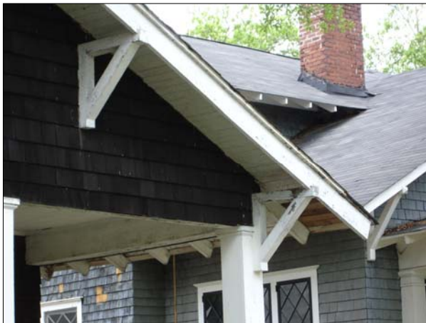
Figure 18: Character defining architectural elements, such as the overhanging roofs and exposed rafters on a bungalow, should be preserved.
