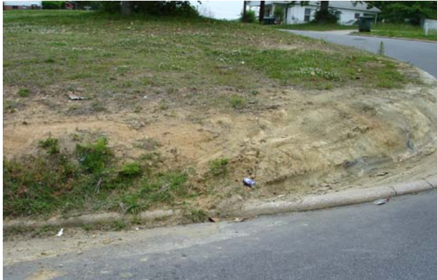
Figure 3: Curb and landscape destroyed by tractor trailers.
