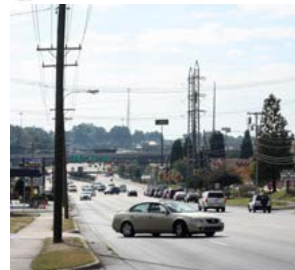
East Innes Looking East From Clay Intersection
