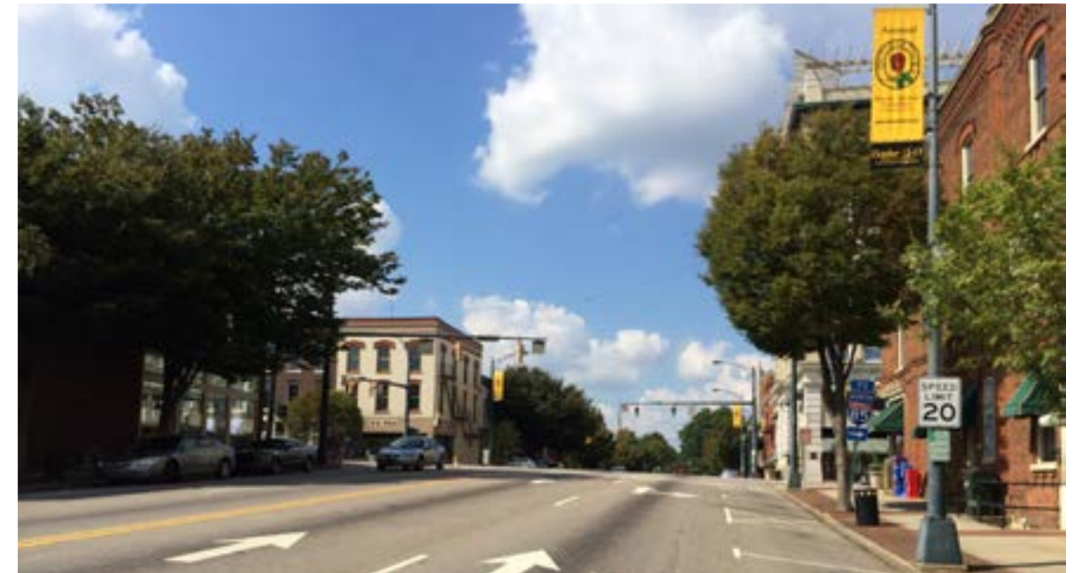
Example of street condition on East Innes in downtown Salisbury
