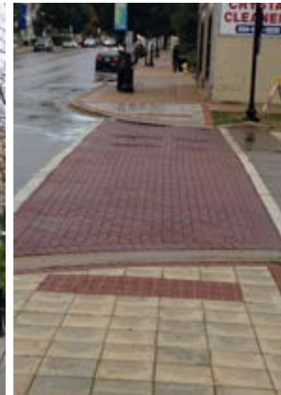
Stamped Asphalt Crosswalk
