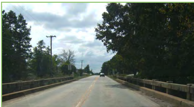
Narrow Bridge over the Southern Railway on Hurley School Road
