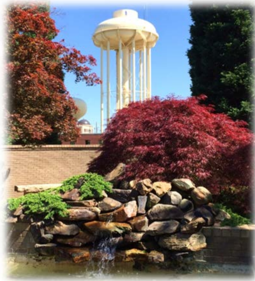
Water and Sewer Water Tower
