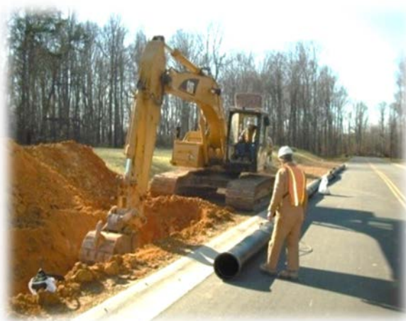
Water and Sewer Construction
