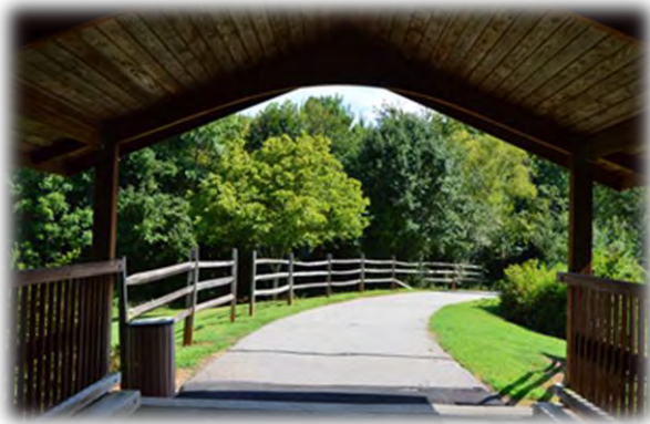
Covered Bridge on Salisbury Greenway
