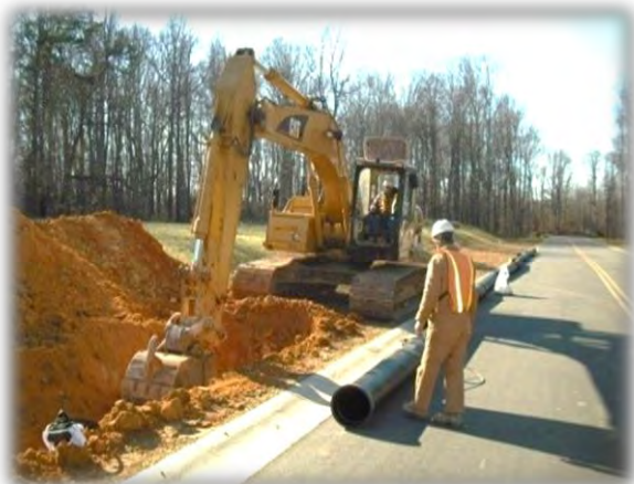
Water and Sewer Construction
