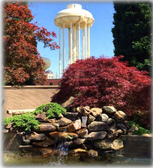
Water and Sewer Water Tower
