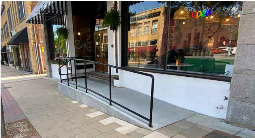
Reversible concrete ramp on commercial storefront
