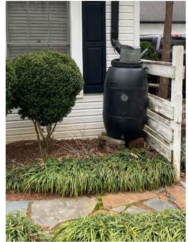
Rain barrel water collection on residential house
