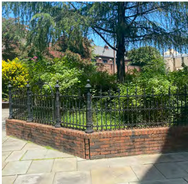
Wrought iron fencing on brick retaining wall
