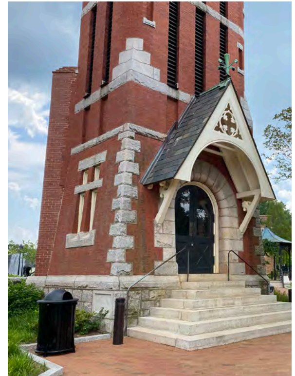
Rusticated granite quoins at the base of the Bell Tower
