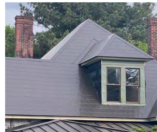
Replacement metal Victorian shingles
