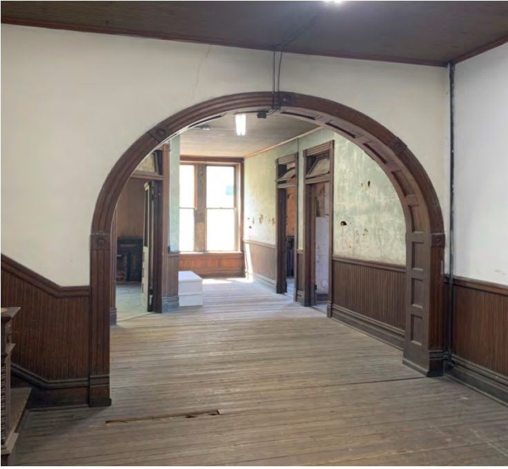
Trim – 4 existing hallway arches retained and repaired,
